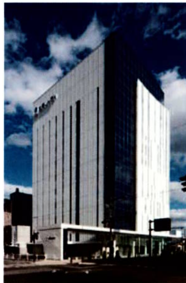
KITAMI SHINKIN BANK, Head Office
